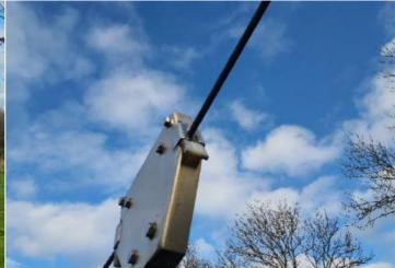
Finding: The nylon inserts are worn or missing at the point Action: Replace worn or missing inserts as required the cable enters the traveller
