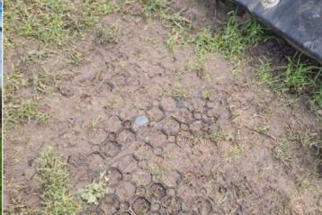
**Finding:** Fixing Pins have been installed in the impact areas **Action:** Remove pins from impact areas of the grass mats
