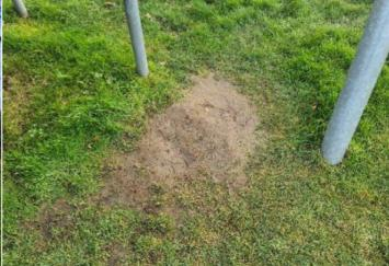
Finding: The grass has eroded within the impact area of the Action: Reinstate the grass or provide an all weather equipment and may not provide the necessary impact attenuating properties for the equipment fall height; the surface may also be slippery in wet weather
