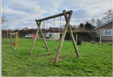
**Finding:** The surfacing width under the seat/s is / are less than 875mm when measured from the centre of the seat outwards, and fail the requirements of BS EN 1176 Part 2
