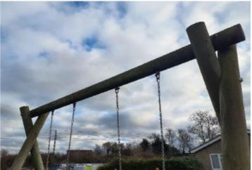
**Finding:** The fixings or components for this item were in excess of 2.5m above the standing surface and could not be recommendations fully accessed by the inspector. We have completed a visual inspection of the fixings from ground level but a maintenance inspection should be undertaken to assess the condition, security and wear of the components at intervals in accordance with the manufacturers recommendations.
