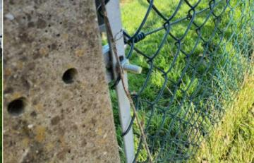
**Action:** Remove excess thread length and deburr or provide cap
