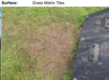
Finding: The grass mats are silted up, the soil is compacted Action: Reinstate as required and the area will become very slippery when the soil is wet.
