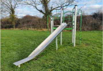
**Finding:** The side of the slide extends less than 500mm above the slide surface at the start section and does not meet the recommendations of BS EN 1176 Part 3
